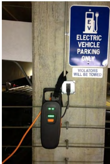
Coca-Cola employee straps up own EVSE to keep it off floor.
